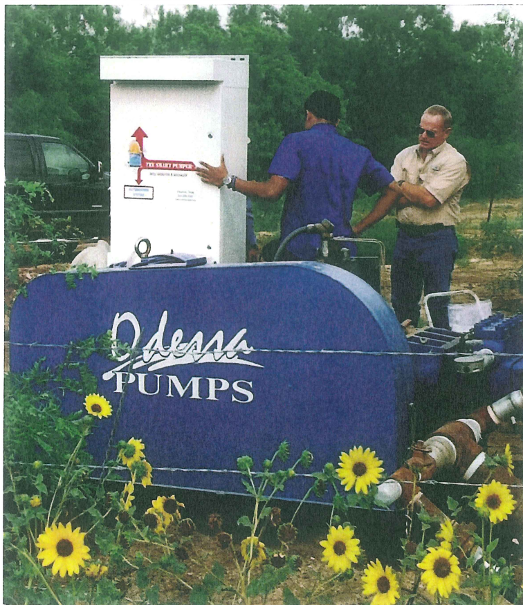
A Smart Pumper automation system for a 70-hp saltwater disposal facility was installed in the Eagle Ford shale. The Smart Pumper intuitively determines injection rate to match tank inflow from multiple wells for continuous precision pumping while maintaining the specific preset tank level.
